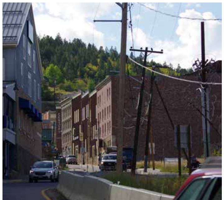
Overhead power and data lines distract from historic district setting
