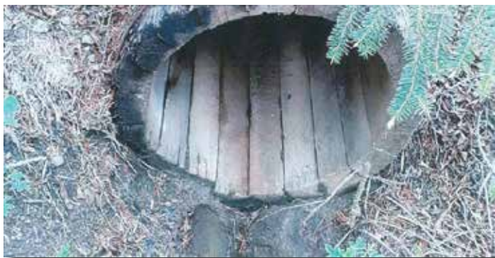
An oak drain pipe in use illustrates the need to modernize infrastructure
